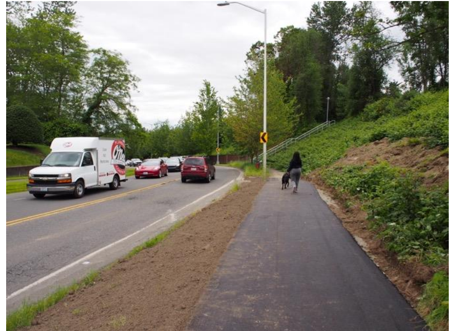
This new walkway on Sylvan Way SW was a previously unselected NSF project delivered as part of the Reconnect West Seattle program
